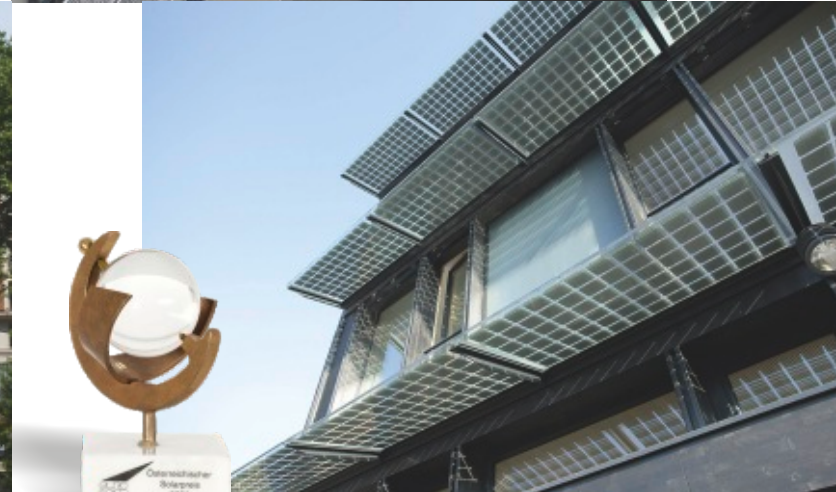
Sunways GAITA Solaire, Paris Modules: 18 ESG, Surface: 32 m 2 , Performance: 3,2 kW p
