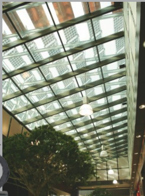
Hypermarchés E.Leclerc, Albi Client: GDF Suez · Construction de la façade: INEO Modules: 1.650 VSG 6/6 en 4 types Dimensions: max. 916 x 1.460 mm Performance: 200 kW p
